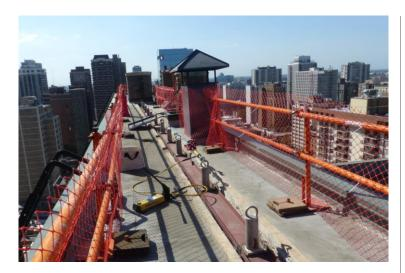
The 1120 North Lake Shore Drive Building is a 20-story mass-masonry residential building completed over 90 years ago in 1925. The building features patinaed standing seam copper gable roofs, setback terraces, and a narrow low slope roof supported by original structural steel, hollow clay tile, and a topping slab. The low slope roof is parallel to Elm Street, and a gabled attic on the east elevation is parallel to Lake Shore Drive; forming the building's L-shaped footprint.
